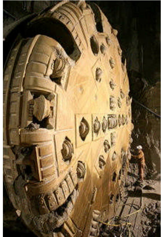
Fig 22:(right) Epping to Chatswood Railway – 7.2 m Diameter TBM Cutterhead
