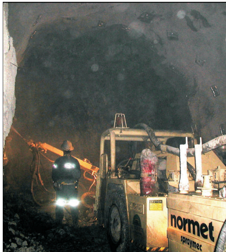
Fig 14: Hydrosaling in Progress 17 .
