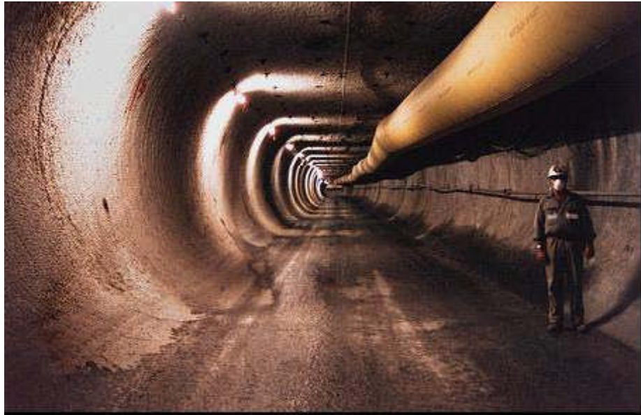
Fig 41: Decline at Broken Hill Mine Driven by the Robbins Mobile Miner, MM130 49
