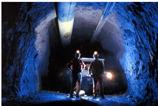
Fig 4: A Development Drive in the Enterprise Section, Mt Isa Copper Mine, Mt Isa, Qld (photo courtesy of www.mining-technology.com ).
