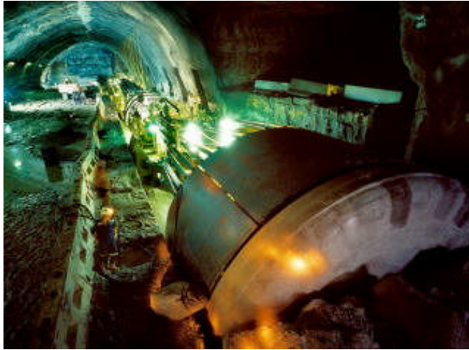
Fig 21:(above) Epping to Chatswood Railway – TBM and Associated Structure
