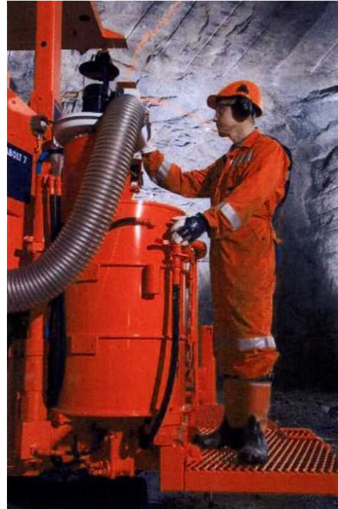
Fig 11: On-board Cementitious Grout Mixing and Pumping System.
